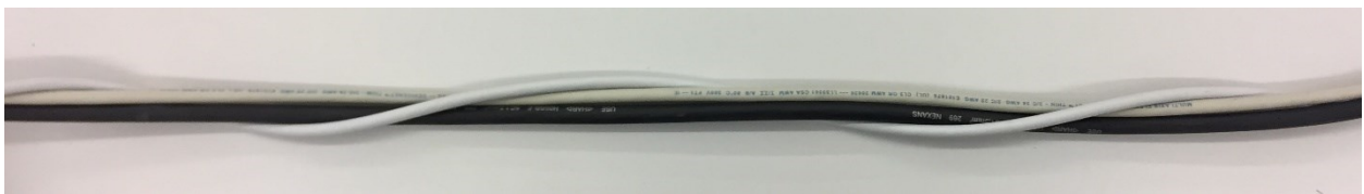
Figure 27: Cable routing, DMX: grey, mains: white, interference source: black, Source: own photograph
