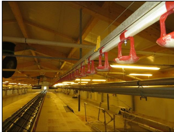
Fig. 59: Drinking water supply line, Source: Own illustration
